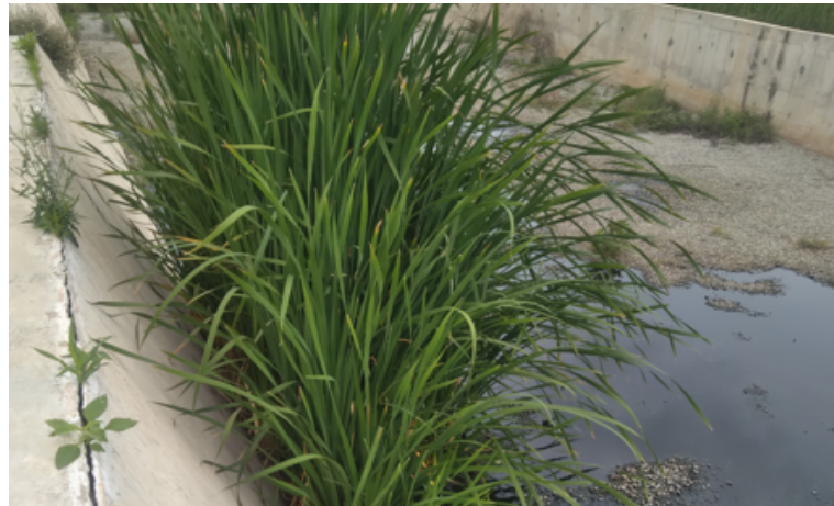
Figure 2: Wastewater on top of substrate as a result of clogging
